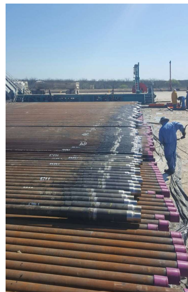
Figure 1. Pre-bucked Bowhead II valves to casing joints.
